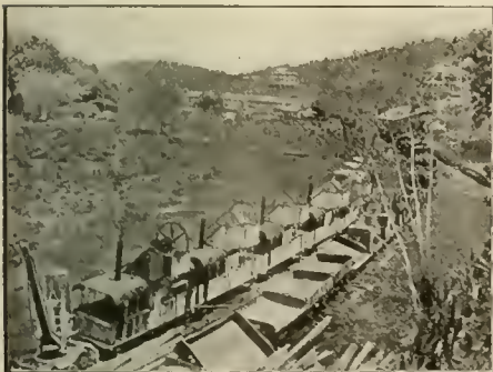
OLD FRENCH MACHINERY ON THE CANAL ZONE.
